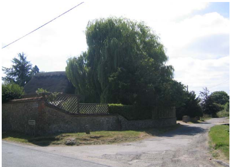
Fig. 61. Triangle Cottage and the track to Slade End Nursery
